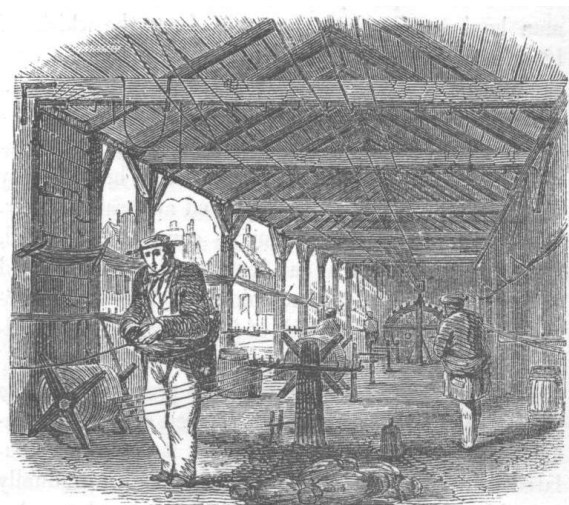
Fig. 1899. SPINNING ROPE YARNS.
