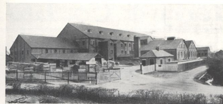
ONE OF OUR WORKS AT BRIDGWATER
