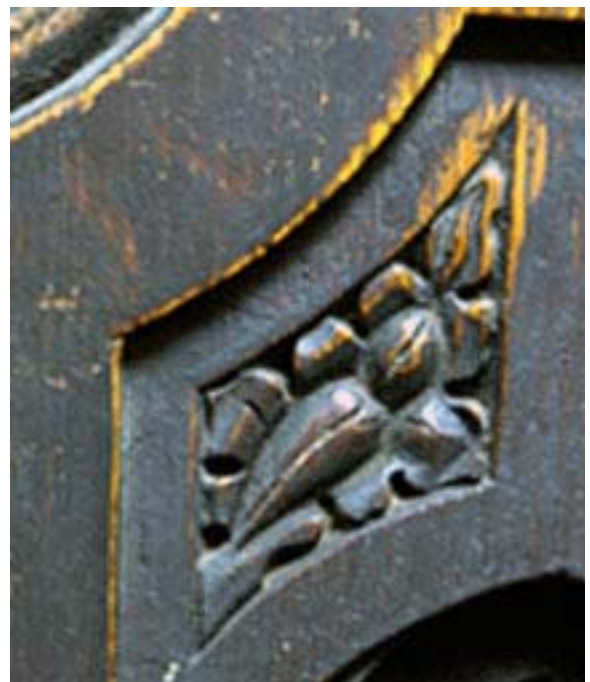
Fig. 34. Variations in the detail of the acanthus-carved spandrels indicate hand-finish and perhaps the work of different carvers. Photographs by Dr Peter Cattermole.
