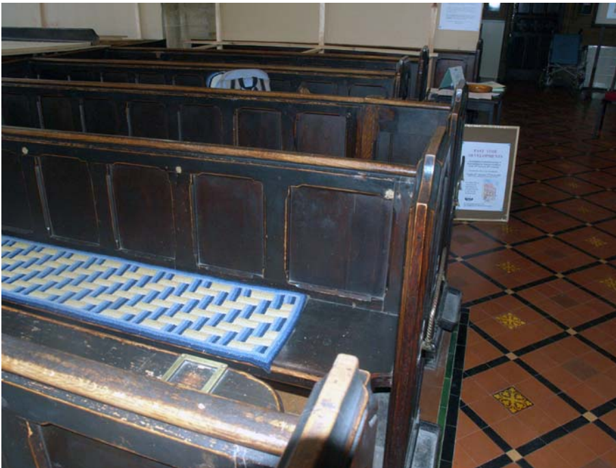
Fig.30. The wider panel of the seat back on the right hand side is part of the evidence for shortening the benches in 1878.
