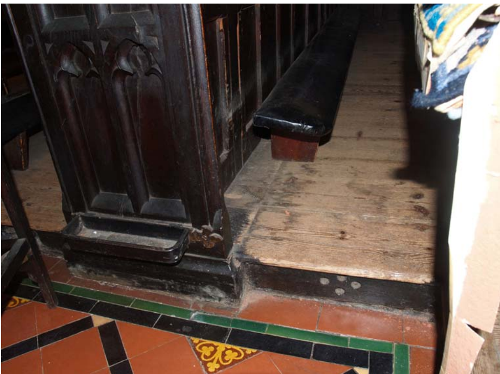
Fig.23. The boarded floor to one of the blocks of benches showing its neat relationship with the 1878 tiling.
