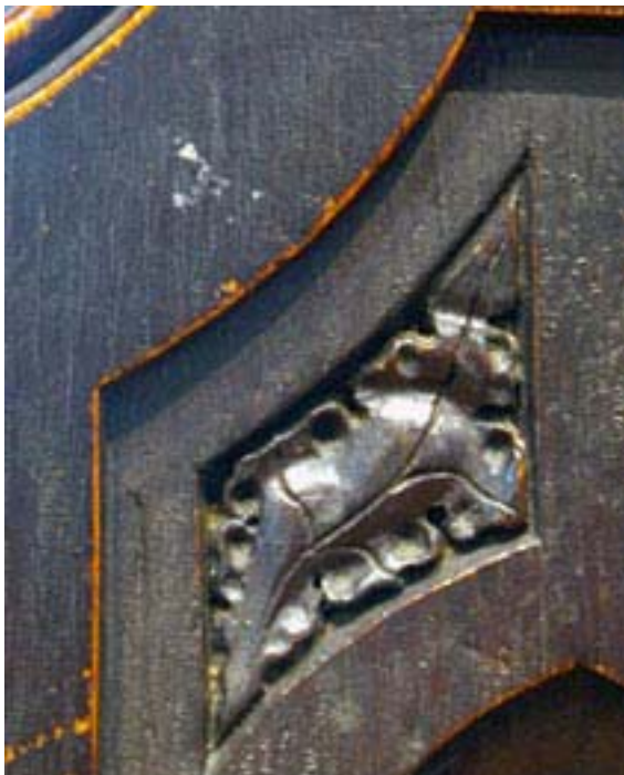
Fig. 34. Variations in the detail of the acanthus-carved spandrels indicate hand-finish and perhaps the work of different carvers. Photographs by Dr Peter Cattermole.
