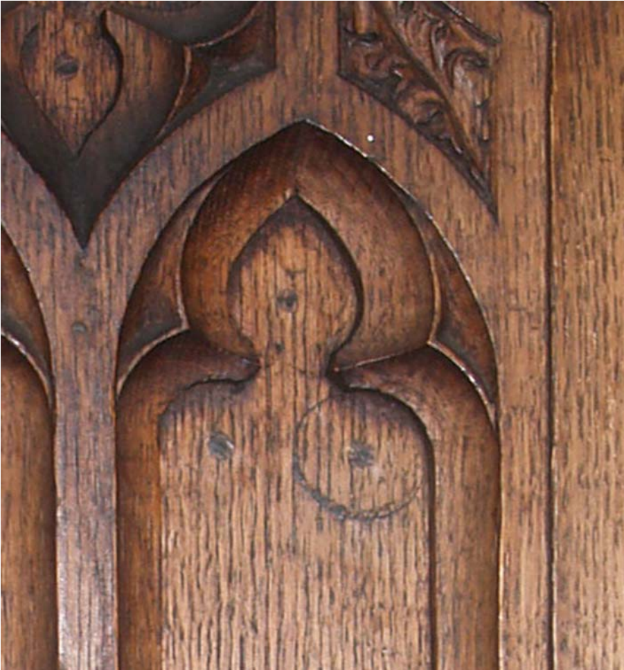
Fig.33. The evidence for machine carving noticed on a bench that has been stripped of its varnish.
