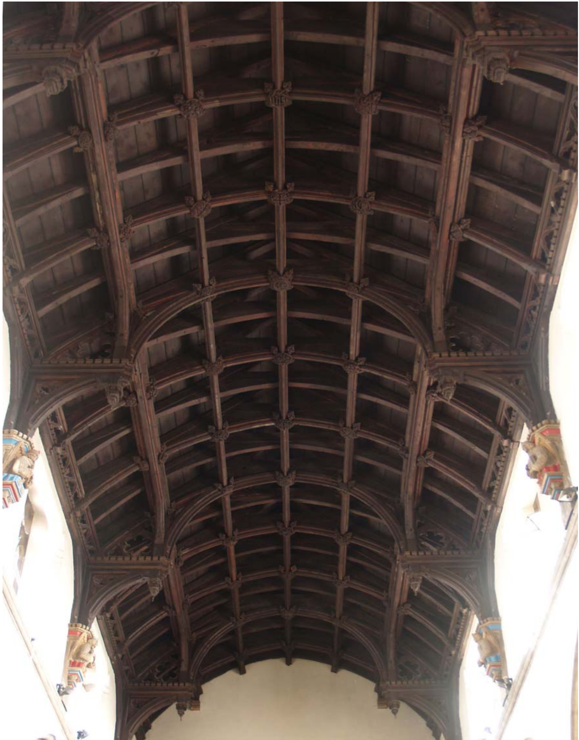
Fig.14. Brakspaar's nave roof incorporating re-cycled timber.
