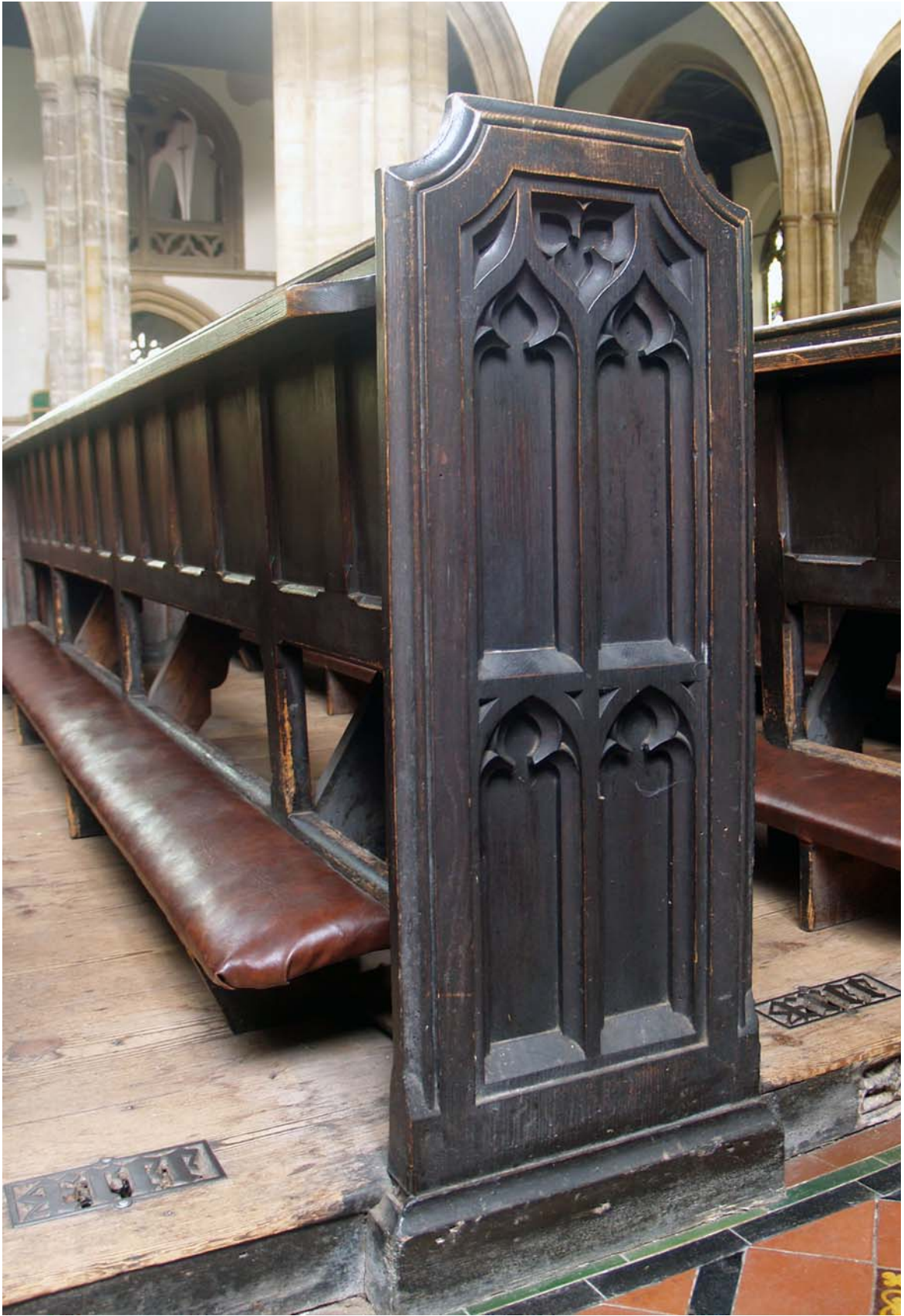
Fig.24. A bench with a type two end showing the construction of the seat back.
