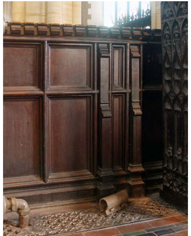
Fig.26. The panelling along the back of the east block benches, defining the cross alley.
