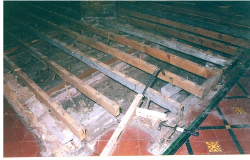
Fig 5 Bearers and joists under the pews in the south block
