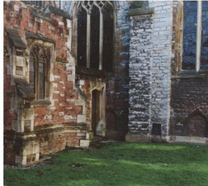
Fig 1 Vents low in the east wall of the Transept
