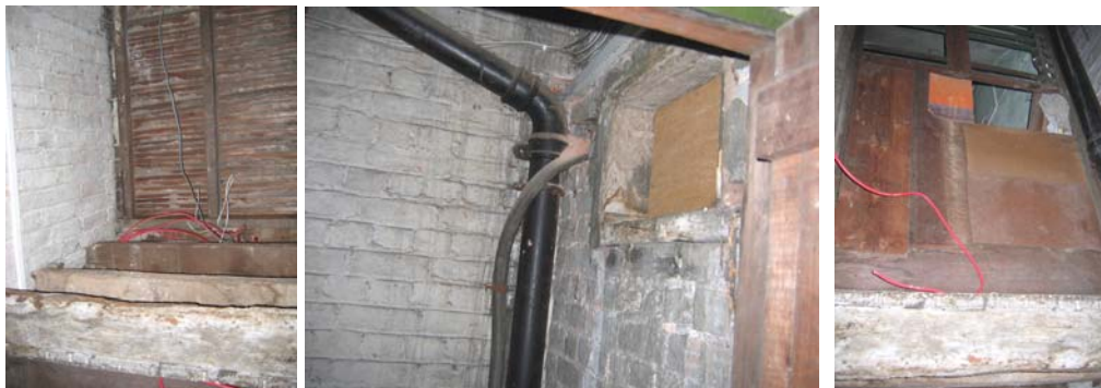
Void beside staircase and panel of attic room above
