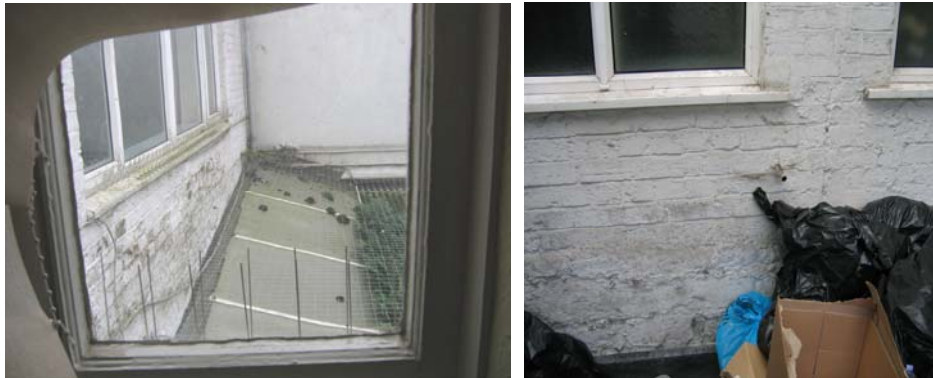
Looking W; South wall
