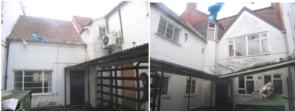
Looking N; Looking SE
