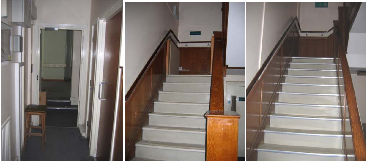
1F-01; Staircase S1
