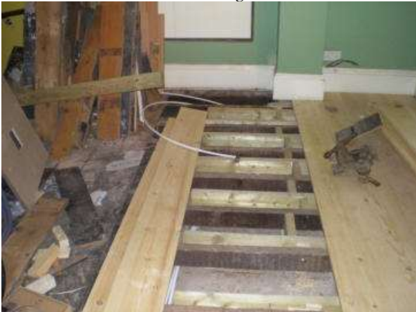
New floorboards being laid
