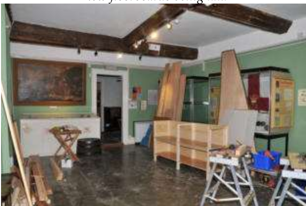
Dismantling the Monmouth room
