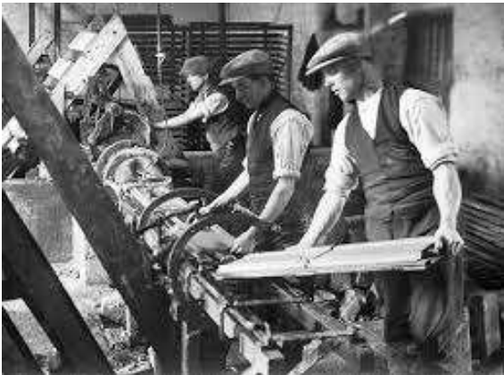
Mechanised tile making
