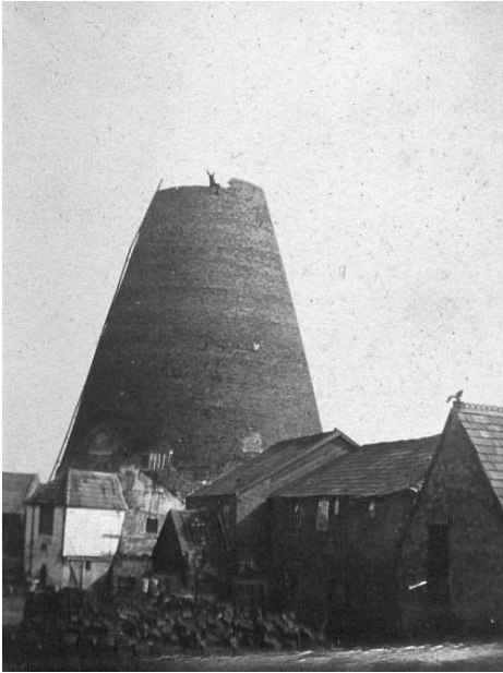
Demolishing the Glass Cone, 1942
