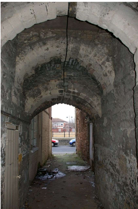
View to the river through the Watergate
