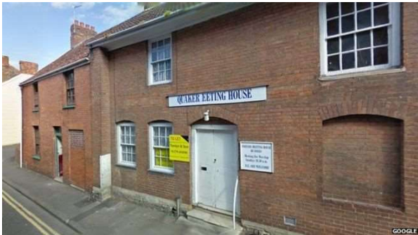
The Quaker Meeting House, Friarn Street
