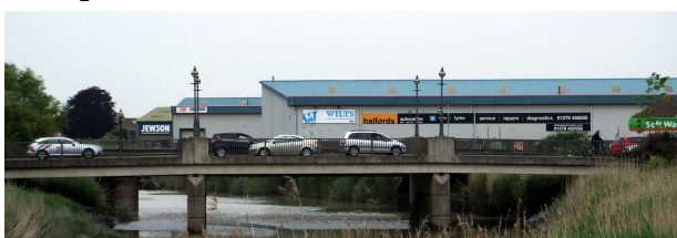
Chandos Bridge, opened 1988
