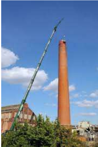
Demolishing the chimney stack
